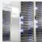
Connectivity and Data Rooms
